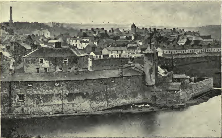
THE KEEP OF ENNISKILLEN CASTLE at present, showing in the outer walls the difference between the ancient and modern masonry. (See page 193.)
